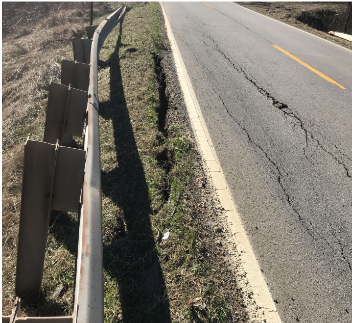
PHOTO 1 Description Approach edge of roadway has erosion up to edge of asphalt and base failure and possible erosion under roadway.
