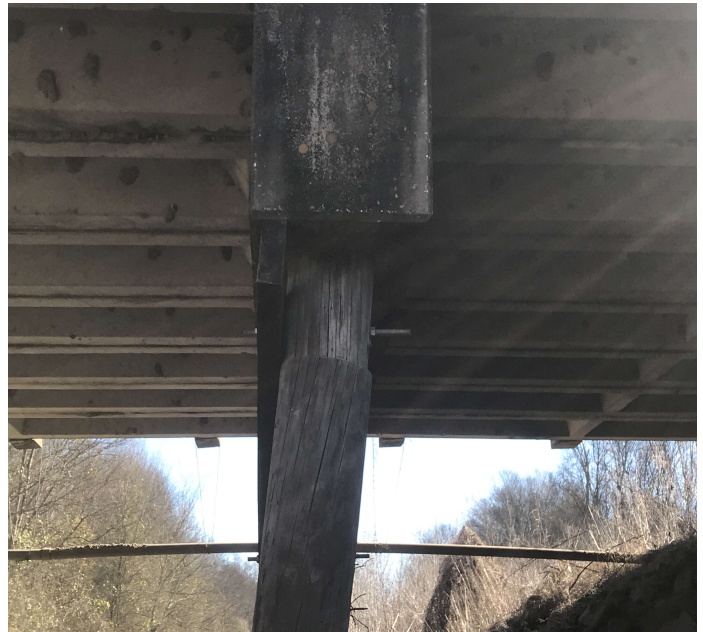
PHOTO 2 Description Bent 2 pile 1 has spliced piece of piling with no collar.
