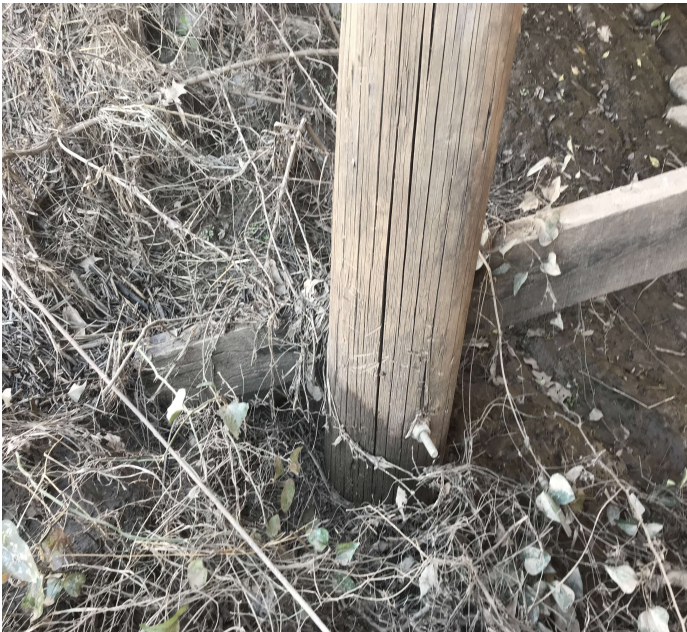
PHOTO 1 Description Bent 4 pile 1 has heavy checking and decay with hollow area near ground line.
