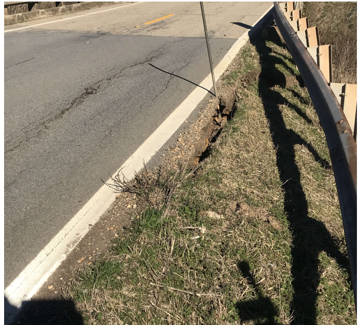
PHOTO 2 Description Approach bent 1 right side slope erosion.
