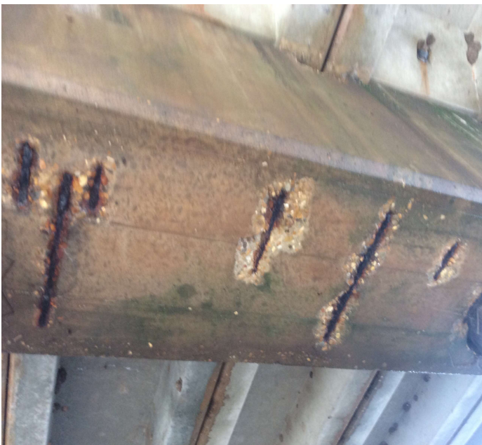
PHOTO 1 Description Cap - Bent 2 bottom face (corrosion)
