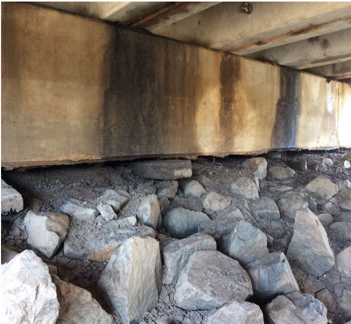
PHOTO 1 Description Endslope - Bent 5 (settlement)
