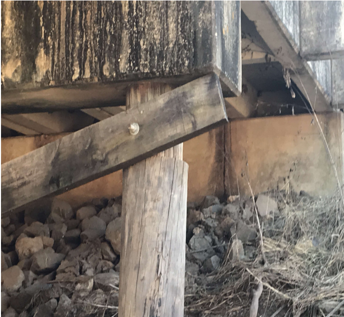
PHOTO 3 Description Bent 2 pile 1 has spliced piece of piling with no collar.
