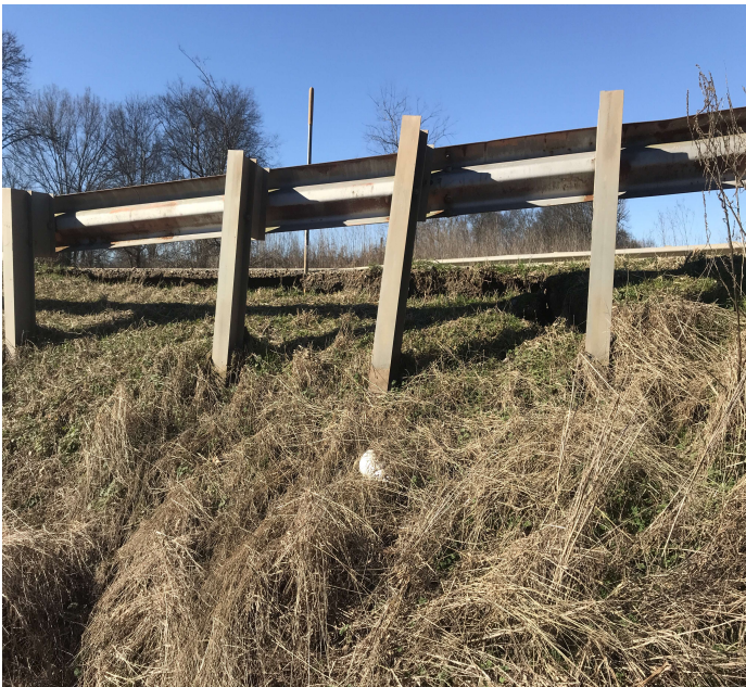
PHOTO 3 Description Approach right side of roadway has material sliding off of shoulder up to roadway.
